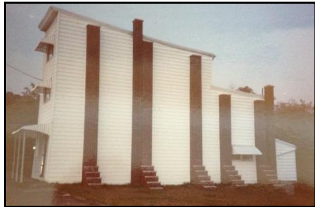
Centralia Row House with brick supports
