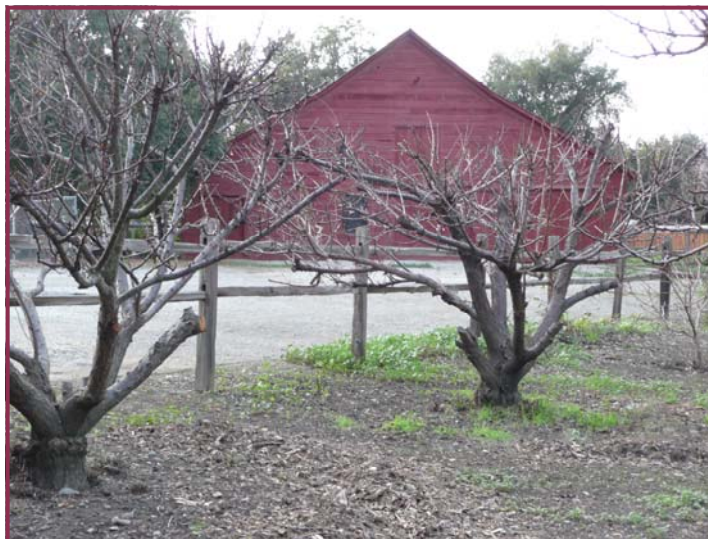
One of two barns located at the back of the Shinn Historic Park and Arboretum. It was salvaged and brought from the Santos' Farm at 1481 Mowry Avenue in Fremont.
